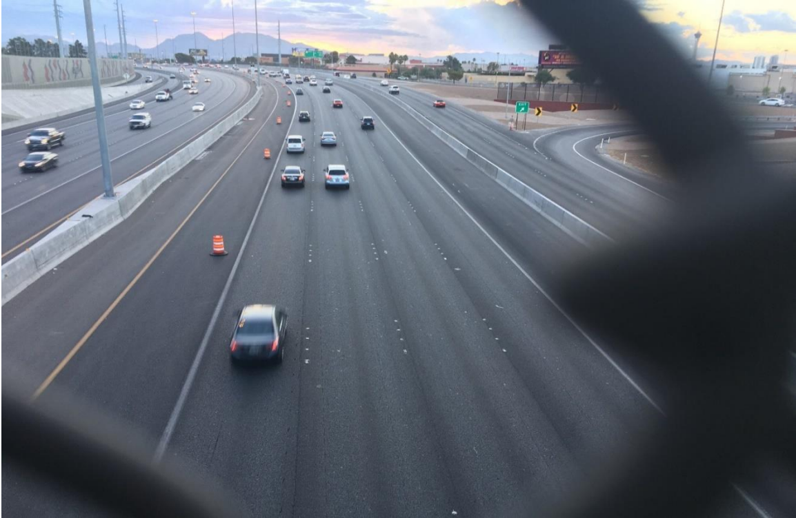
Figure 3-19. Eastbound traffic at Site 5
